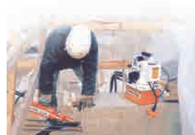
The PE60 used for pre-stressing.
